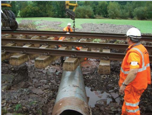
Lifting track to repair drainage pipe. © Network Rail 2015
